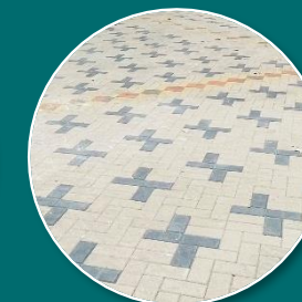
New flooring and improved drainage
