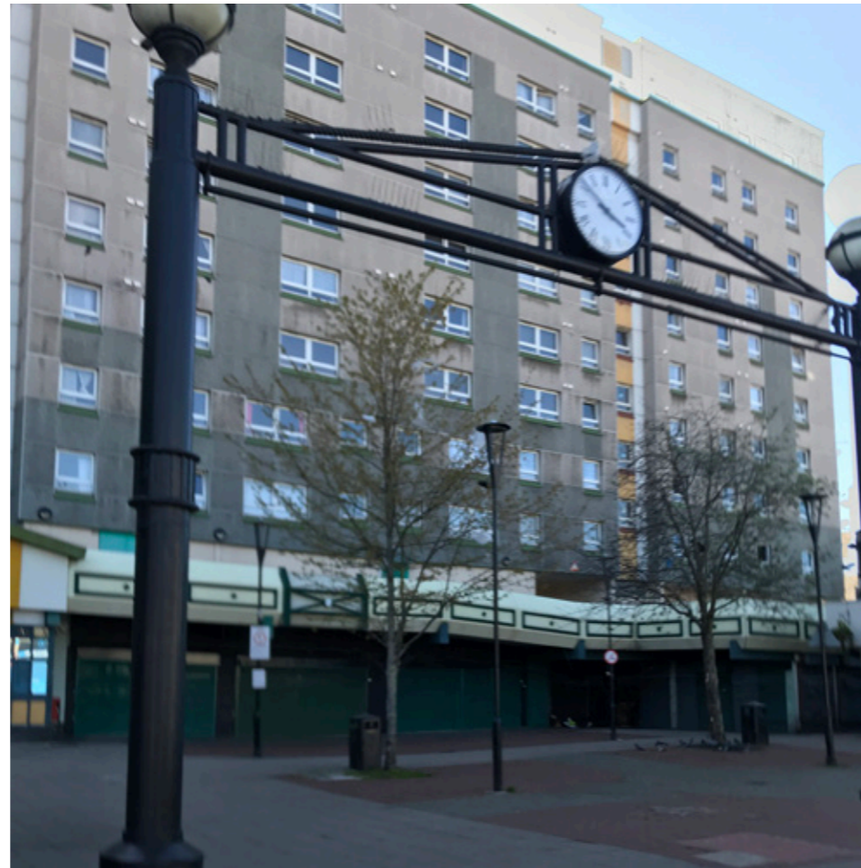
Site Photo: Existing Clock Arch on Queen's Square
