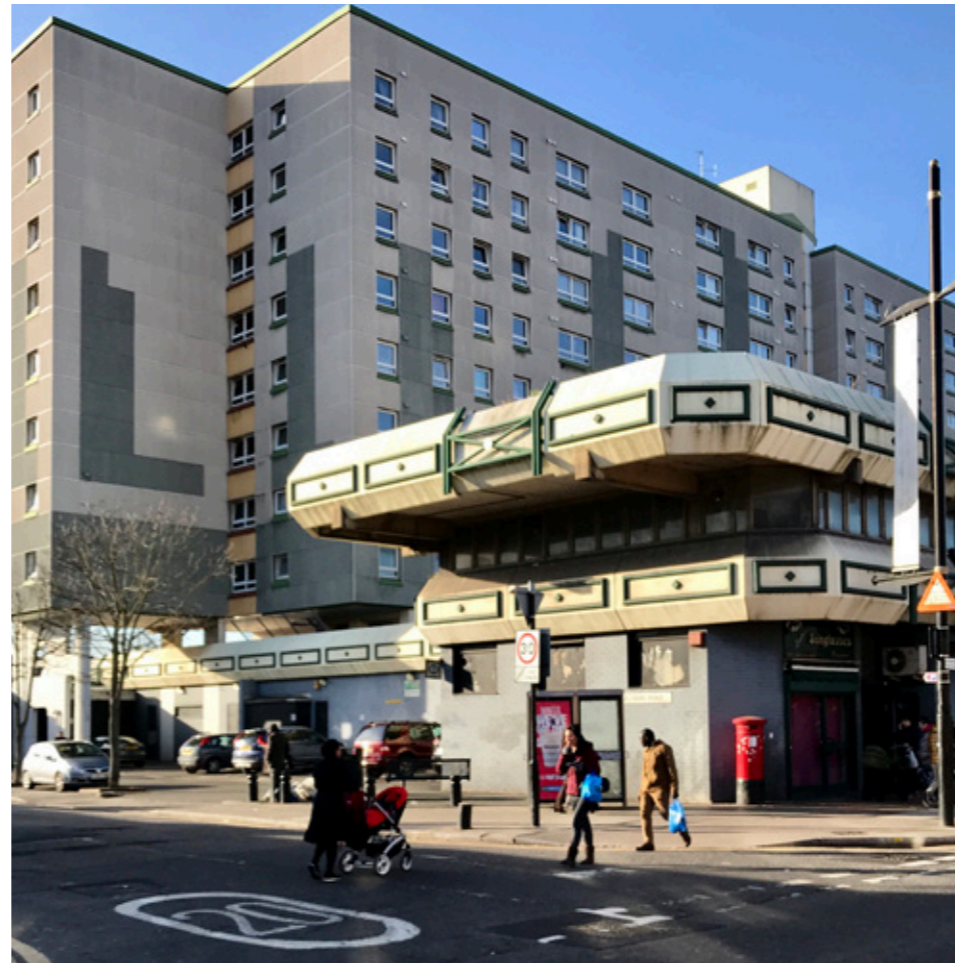
Site Photo: Hamara Ghar Flats
